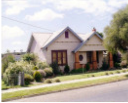
SL 247 - House, 35 Napier Street, STAWELL
