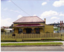
SL 248 - House, 39 Napier Street, STAWELL
