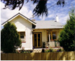
SL 250 - House, 56 Napier Street, STAWELL
