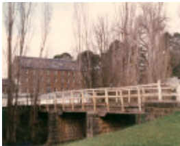
B6920 Andersons Mill Bridge
