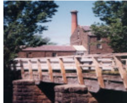
B6920 Andersons Mill Bridge
