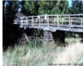
B6920 Andersons Mill Bridge
