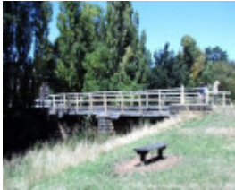
B6920 Andersons Mill Bridge
