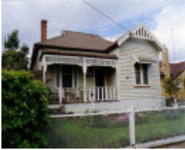
SL 260 - House, 19 Patrick Street, STAWELL
