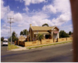
SL 265 - House, 48 Patrick Street, STAWELL
