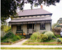
SL 269 - House, 65 Patrick Street, STAWELL
