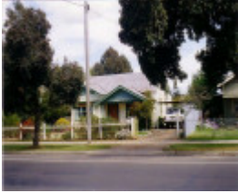
SL 270 - House, 66 Patrick Street, STAWELL
