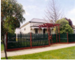
SL 272 - House, 71 Patrick Street, STAWELL
