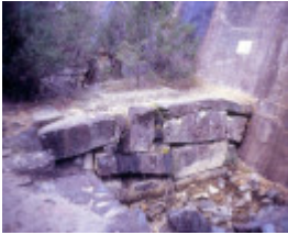
h01556 heatherlie quarry grampians national park halls gapp rock and concrete crane base she project 2004
