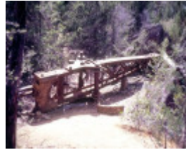
h01556 heatherlie quarry grampians national park halls gapp small jib crane she project 2004
