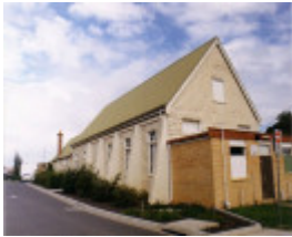
SL 277 -Holy Trinity Anglican Church Parish Hall, Scallan Street, STAWELL
