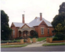
SL 279 - Former Presbyterian Manse, 9 Scallan Street, STAWELL
