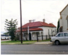
SL 282 - House, 23 Scallan Street, STAWELL
