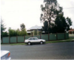
SL 288 - House, 35 Scallan Street, STAWELL
