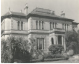
B0492 Oakleigh Hall Te Arai Avenue St Kilda
