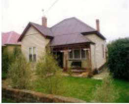
SL 294 - House, 6 Seaby Street, STAWELL
