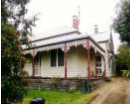
SL 298 - House, 13 Seaby Street, STAWELL
