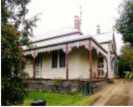
SL 298 - House, 13 Seaby Street, STAWELL
