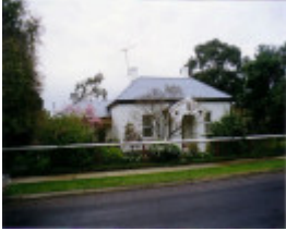
SL 299 - House, 14 Seaby Street, STAWELL
