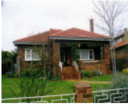
SL 300 - House, 15 Seaby Street, STAWELL
