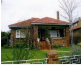
SL 300 - House, 15 Seaby Street, STAWELL
