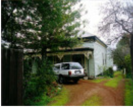
SL 301 - House, 16 Seaby Street, STAWELL
