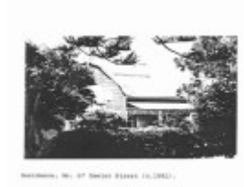
Residence, 67 Gawler Street
