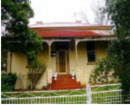
SL 306 -House, 23 Seaby Street, STAWELL
