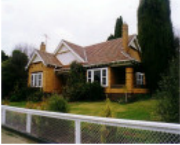
SL 308 - House, 25 Seaby Street, STAWELL
