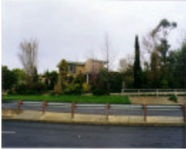
SL 310 - House, 27-29 Seaby Street (corner Stone Street), STAWELL
