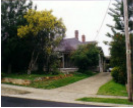
SL 312 - House, 33 Seaby Street, STAWELL
