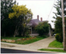
SL 312 - House, 33 Seaby Street, STAWELL
