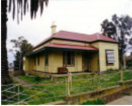
SL 313 - House, 34 Seaby Street, STAWELL
