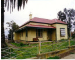
SL 313 - House, 34 Seaby Street, STAWELL
