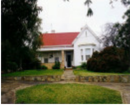
SL 314 - House, 37 Seaby Street, STAWELL
