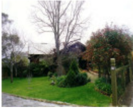
SL 315 - House, 38-40 Seaby Street, STAWELL
