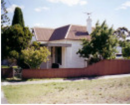
SL 317 - House, 42 Seaby Street, STAWELL
