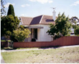
SL 317 - House, 42 Seaby Street, STAWELL
