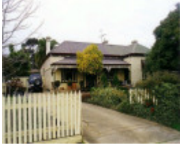
SL 318 - House, 43 Seaby Street, STAWELL
