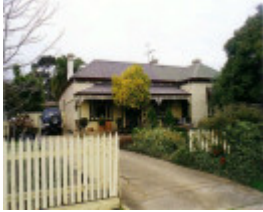
SL 318 - House, 43 Seaby Street, STAWELL
