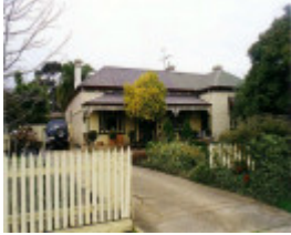
SL 318 - House, 43 Seaby Street, STAWELL
