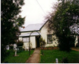
SL 319 - House, 49 Seaby Street, STAWELL
