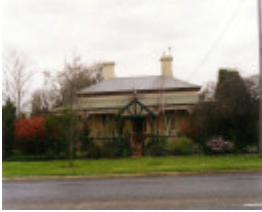
SL 320 - House, 65 Seaby Street, STAWELL
