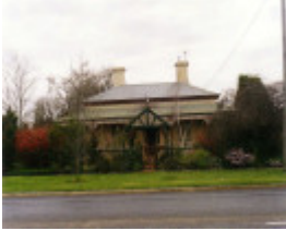
SL 320 - House, 65 Seaby Street, STAWELL
