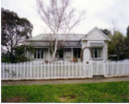
SL 321 - House, 66 Seaby Street, STAWELL
