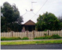
SL 322 - House, 'Dulkeith', 15 Shirreff Street, STAWELL
