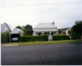
SL 323 - House, 19 Shirreff Street, STAWELL
