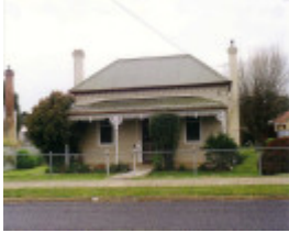
SL 324 - House, 21 Shirreff Street, STAWELL
