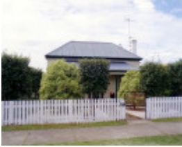
SL 327 - House, 27 Shirreff Street, STAWELL
