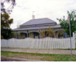
SL 330 - House, 43 Shirreff Street, STAWELL
