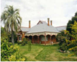
SL 334 - House, 2 Skene Street, STAWELL
