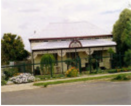
SL 335 - House, 4 Skene Street, STAWELL
