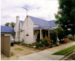
SL 336 - House, 8 Skene Street, STAWELL
