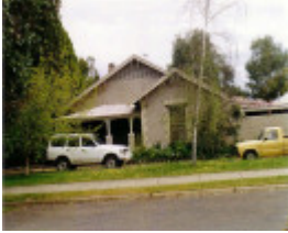
SL 338 - House, 12 Skene Street, STAWELL
