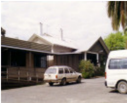
SL 339 - Skene Street Special School, 13 Skene Street, STAWELL
