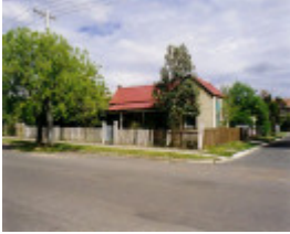
SL 340 - House, 14 Skene Street, STAWELL
