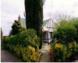
SL 343 - House, 18 Skene Street, STAWELL
