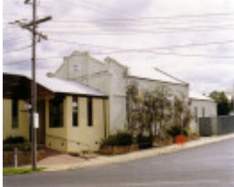
SL 344 - Church of Christ, 18 Sloane Street (corner Skene Street), STAWELL
