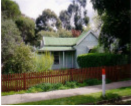
SL 346 - House, 22 Skene Street, STAWELL
