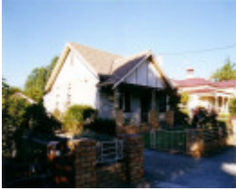
SL 347 - House, 23 Skene Street, STAWELL
