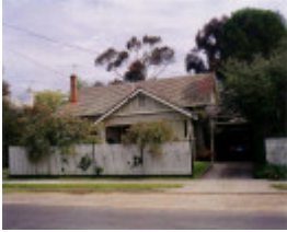
SL 348 - House, 24 Skene Street, STAWELL
