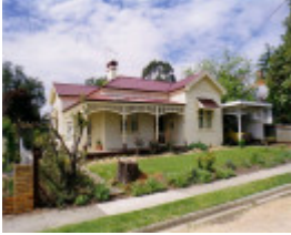
SL 349 - House "Bronwyn", 25 Skene Street, STAWELL
